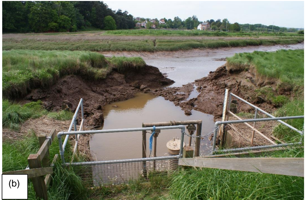
Figure 5.3 Regulated tidal exchange scheme at Goosemoor: (a) sluice structure facing into the estuary and (b) culvert and stop logs inside the site
